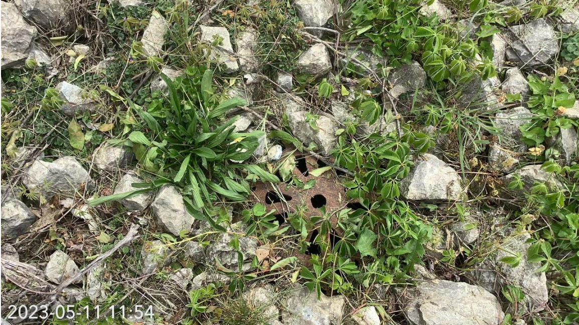
Photograph Location 5. Representative view of existing culvert/storm drain within the Project area.
